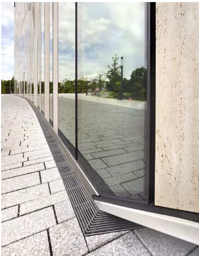
On the left: Façade channel FR-10K fully made of stainless steel
