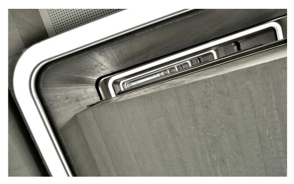
View of the tunnel: Along the ceiling openings above the eye of the stairs a crown of light using powerful LED modules has been created on all eight floors.
