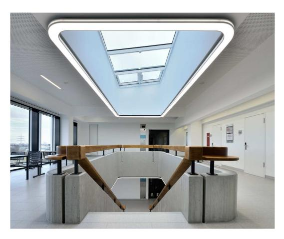
The coverings of satin acrylic glass runs softly round the opening in the ceiling to provide even and diffuse lighting.
